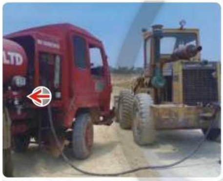
Mobile Diesel Refueling India Cements, Dalavoi
